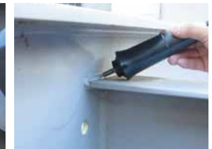
Measuring the strength of welding sections (Checking tension strength)
